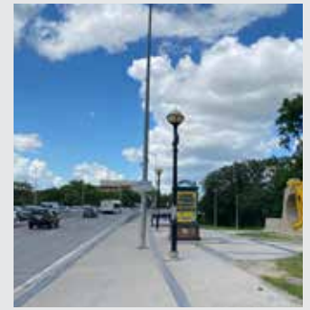
Looking North over bridge
